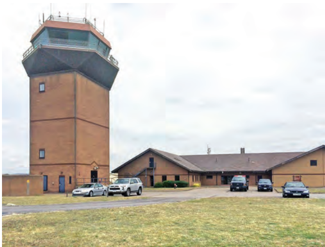
The modern RAF Lakenheath control tower, the adjacent building houses the Radar Approach Control. Photo Keith Ward
